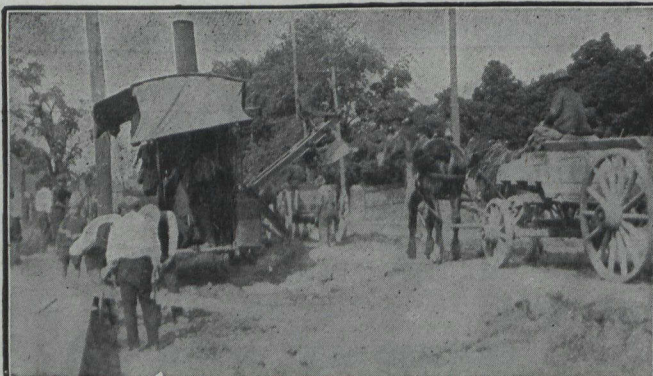
Road Grading with a Keystone—The Skimmer Scoop is employed.
