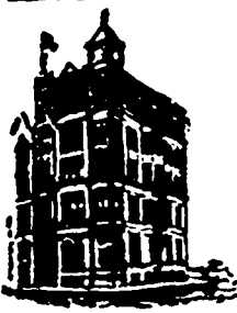
HEAD OFFICE BUILDING, MONTREAL.
