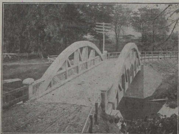
Middle Road Bridge, 80-ft. Span
