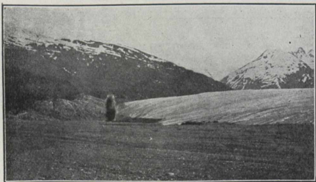
Blasting New Channel for Underground Streams at Foot of Spencer Glacier.
