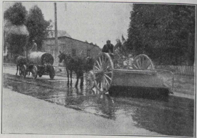
Sprinkling and Spreading Bitumen
