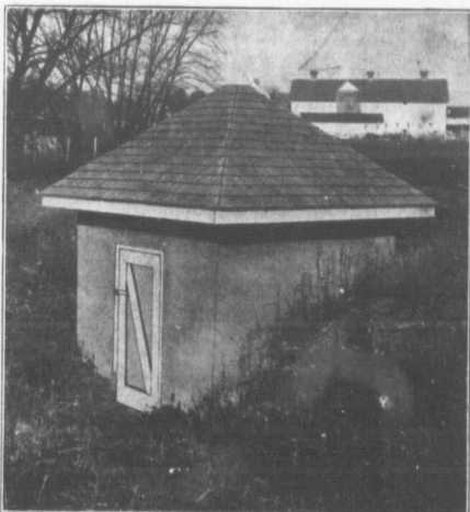
A Suitable and Permanent Home for the Hydraulic Ram
