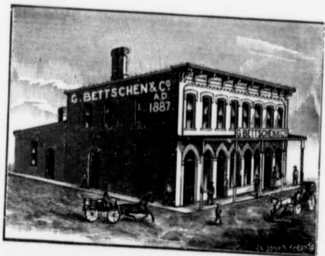
Bettschen's Block, Front Street, New Dundee, Ontario. Built 1887 by G. Bettschen.
