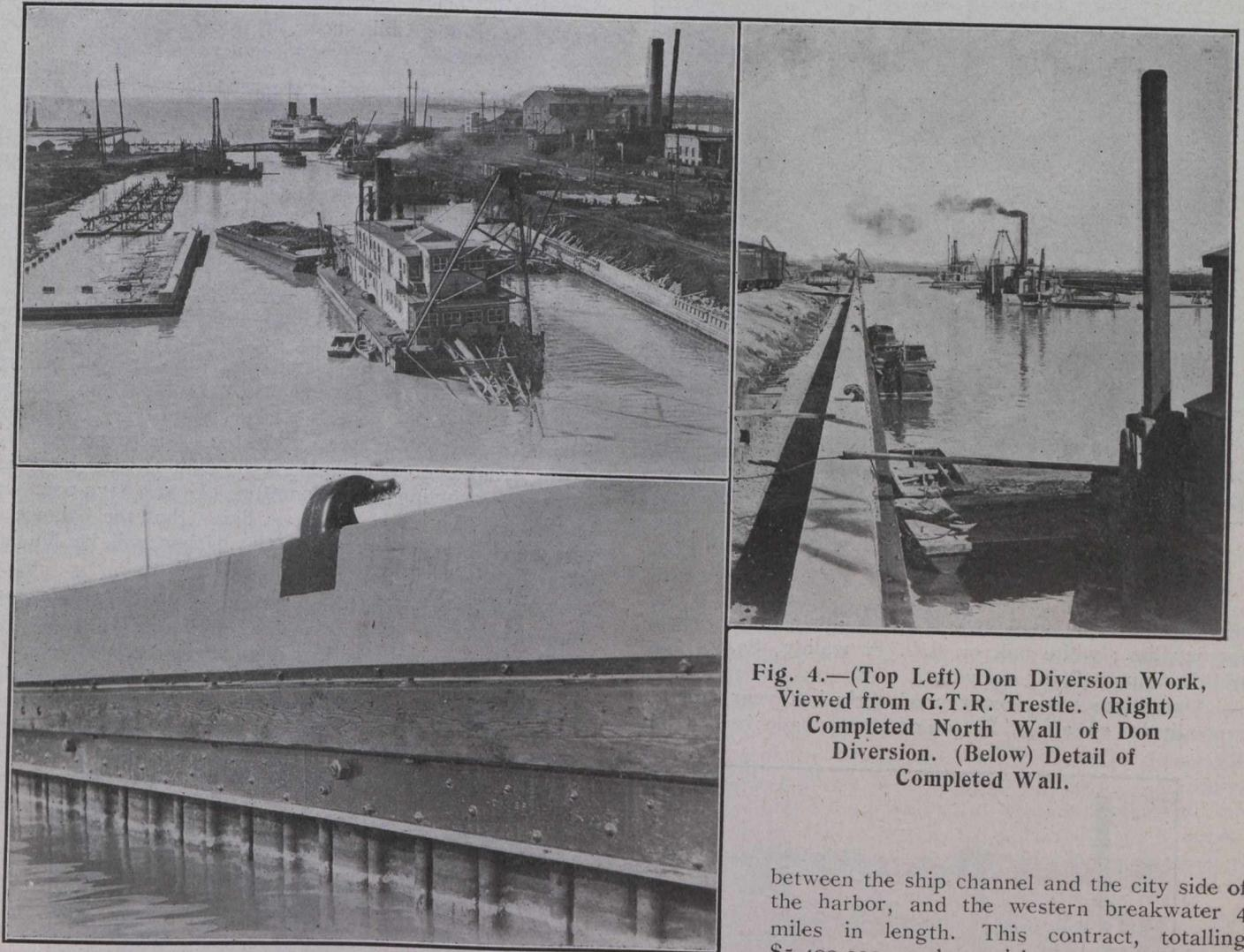
Fig. 4.—(Top Left) Don Diversion Work, Viewed from G.T.R. Trestle. (Right) Completed North Wall of Don Diversion. (Below) Detail of Completed Wall.
