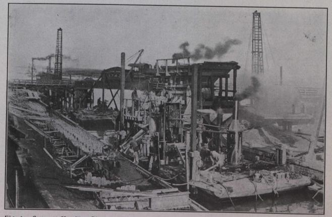
Fig. 1.-Concrete Handling Plant at Work on Don Diversion Channel Walls, Toronto Harbor Commission.
