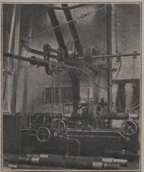
Crane for Mounting Axles in Axle Lathe.
