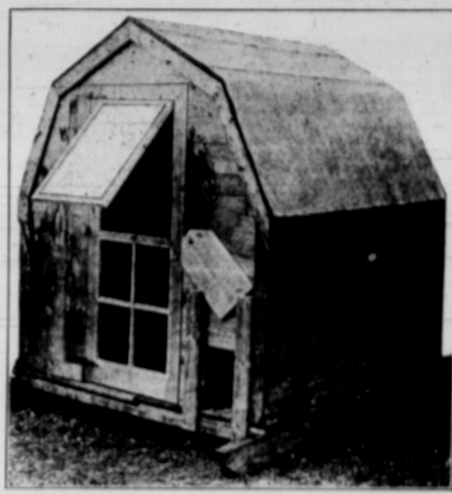
A cheap portable colony house for rearing chickens, made out of two piano boxes.
