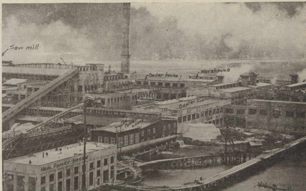
Quite a contrast to the mill at Portneuf is the extensive plant at Ocean Falls, B.C. The mountain comes so close to the sea that at most of the mill is built on piles. All communication with this mill is by boat or wireless.
