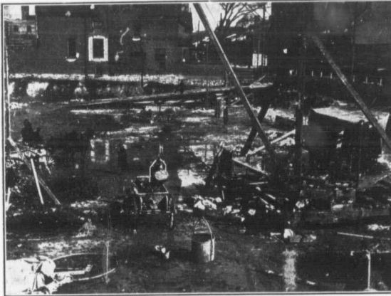
BUILDING THE NEW BOOK ROOM.
