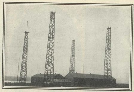
General View of the Marconi Stations at Glace Bay, N.S.-Receiving and Transmitting Towers and Condensing Station.
