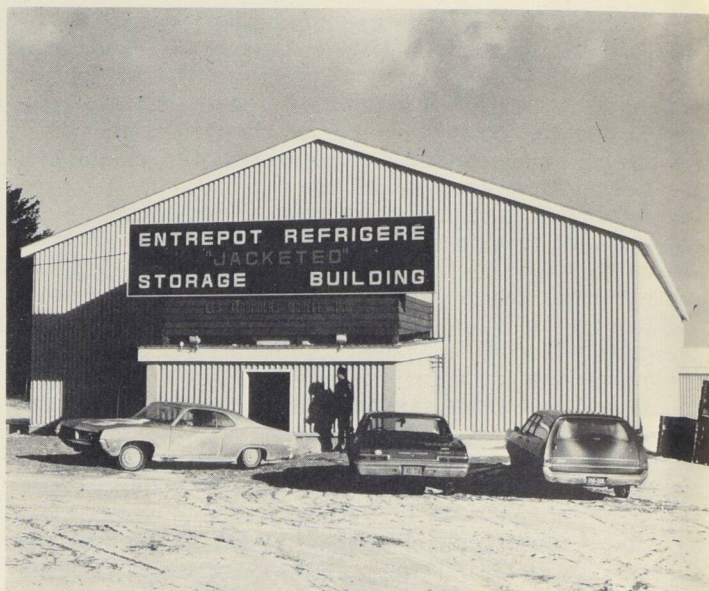
Jacketed storage building used to store carrots at Sherrington, Quebec.
