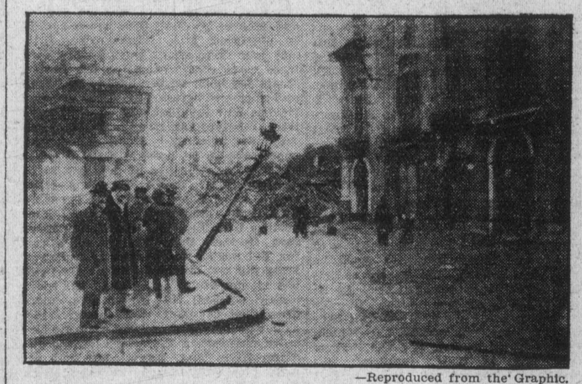
The wreckage in Via Canour, one of the main streets of Messina.
