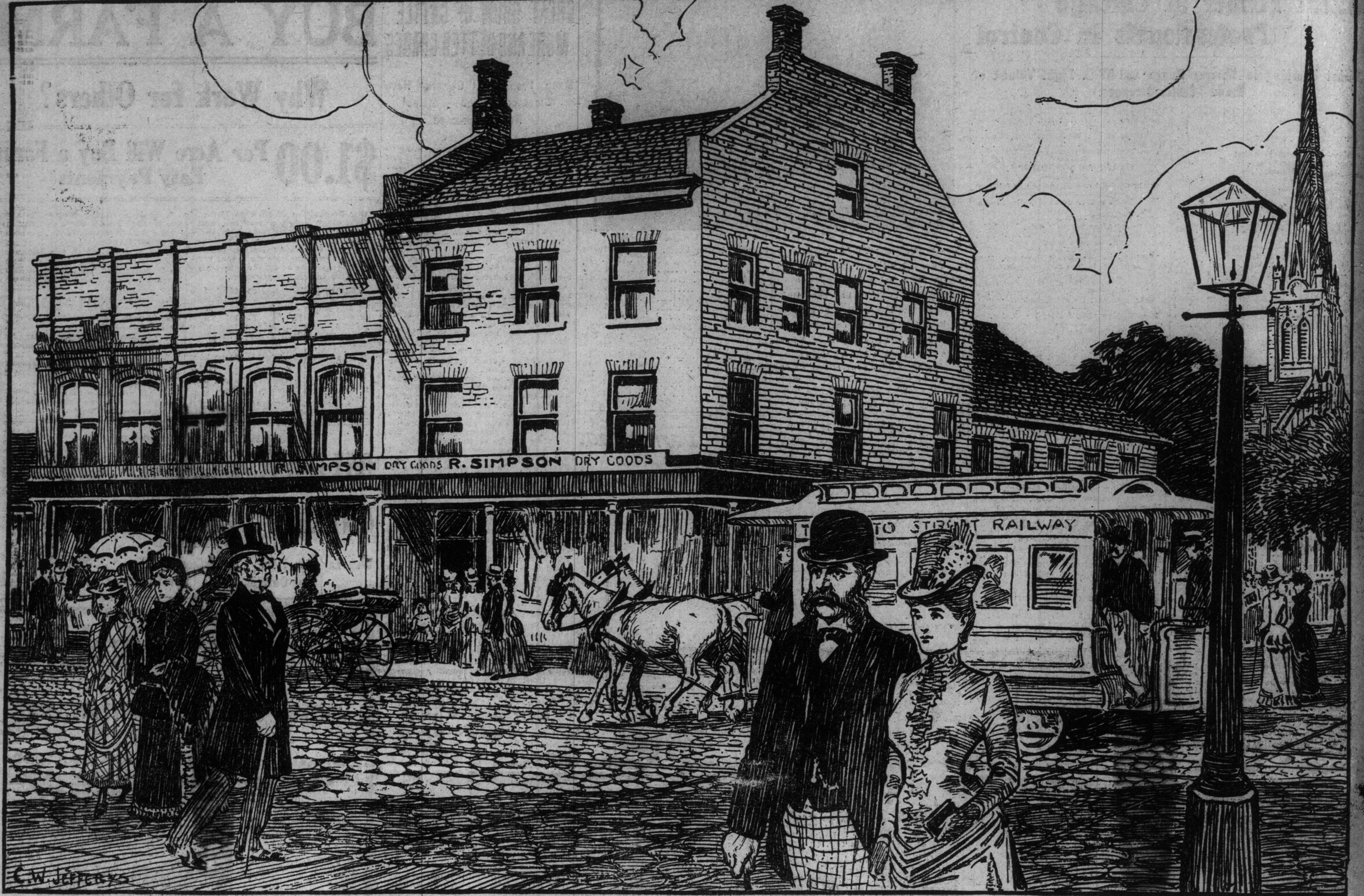
No. 6.—The Red Brick Store of Robert Simpson, Esq., Corner Yonge and Queen Streets, Toronto, Canada, 1882.
