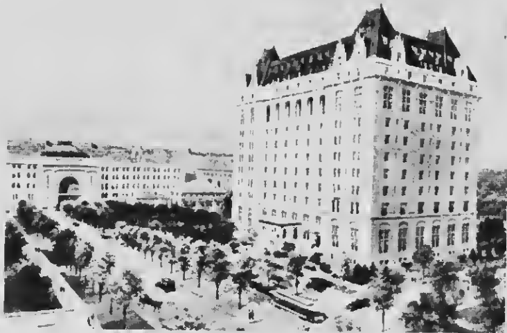
Winnipeg Union Station
