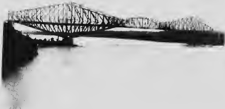
The Quebec Bridge
