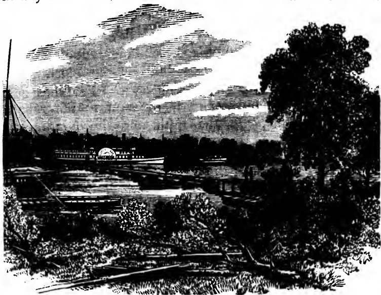
PONTOON BRIDGE AT DEEP BOTTOM.
