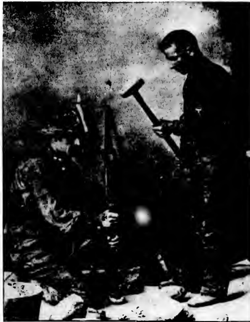
MINERS ENGAGED IN HAND DRILLING.
