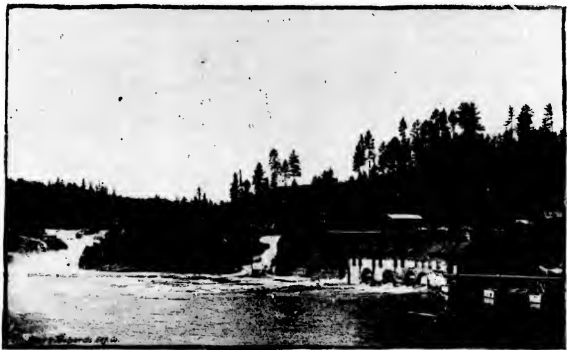
HYDRAULIC WORKS AND AIR COMPRESSORS—MENOMINEE RIVER.
