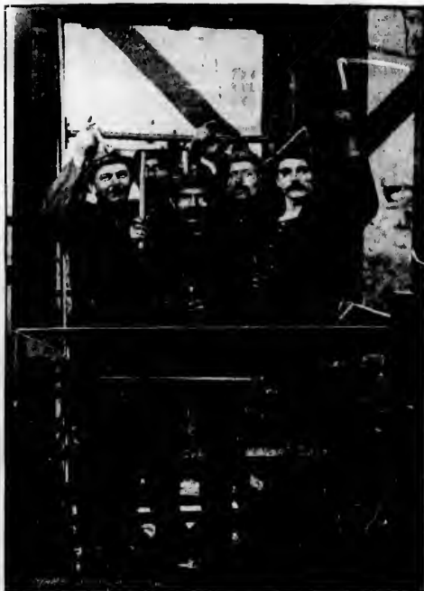
MINERS DESCENDING SHAFT, PEWABIC MINE.
