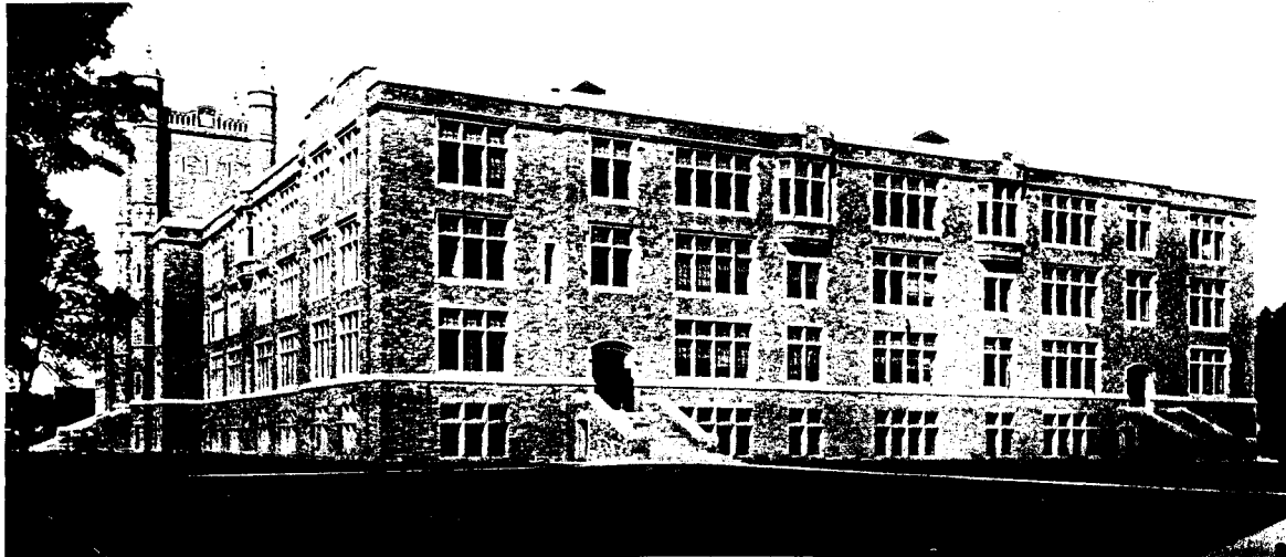
Central Technical School, Toronto, Can. Concrete Floors laid by Master Builders Method. Ross & Macdonald, Architects. Success Brothers, General Contractor.
