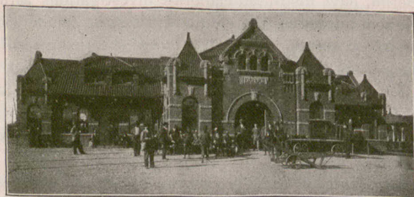
UNION DEPOT AT DALLAS, TEXAS, ROOFED WITH MERCHANT'S METAL "SPANISH" TILES.
