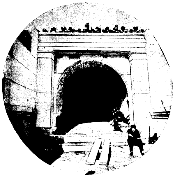
TUNNEL EXTENDING UNDER THE STADE THROUGH WHICH ATHLETES ALONE WERE ADMITTED.
