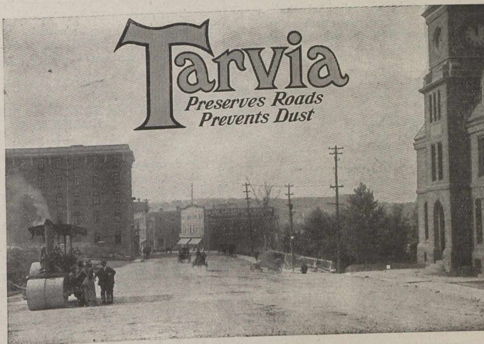
Racine Street, Chicoutimi, Quebec. Road constructed with "Tarvia-X."
