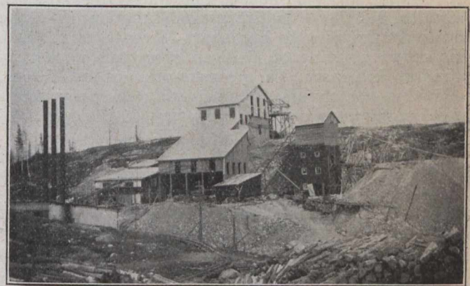
Power plant, Mill, and No. 1 Shaft. All dumps to left of shaft are Concentrating Ore.
