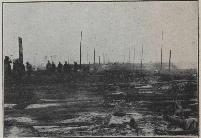
Golden Avenue After the Fire.
