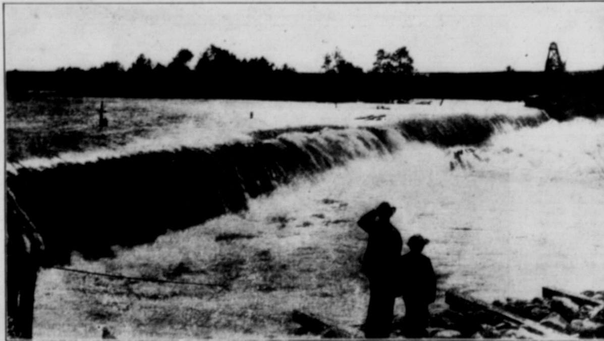
Irrigation in the Province of Alberta—Dam Across the Bow River. This Ensures a Constant Head of Water for One of the Big Irrigation Ditches of Southern Alberta.
