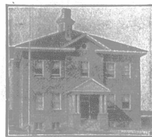
House built in New Liskeard of blocks made by the London Face-Down Block Machine
