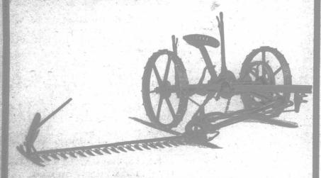
It is made in four sizes, cutting 41, 5, 6 and 7 feet, respectively.
