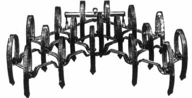
Away ahead of all others; all steel frame; no wood to decay and wear out; lightest draught spring tooth harrow made; teeth quickly adjusted—only one nut to loosen; will not clog or bury. On stony land its work is perfection; in sticky ground there is none like it.
