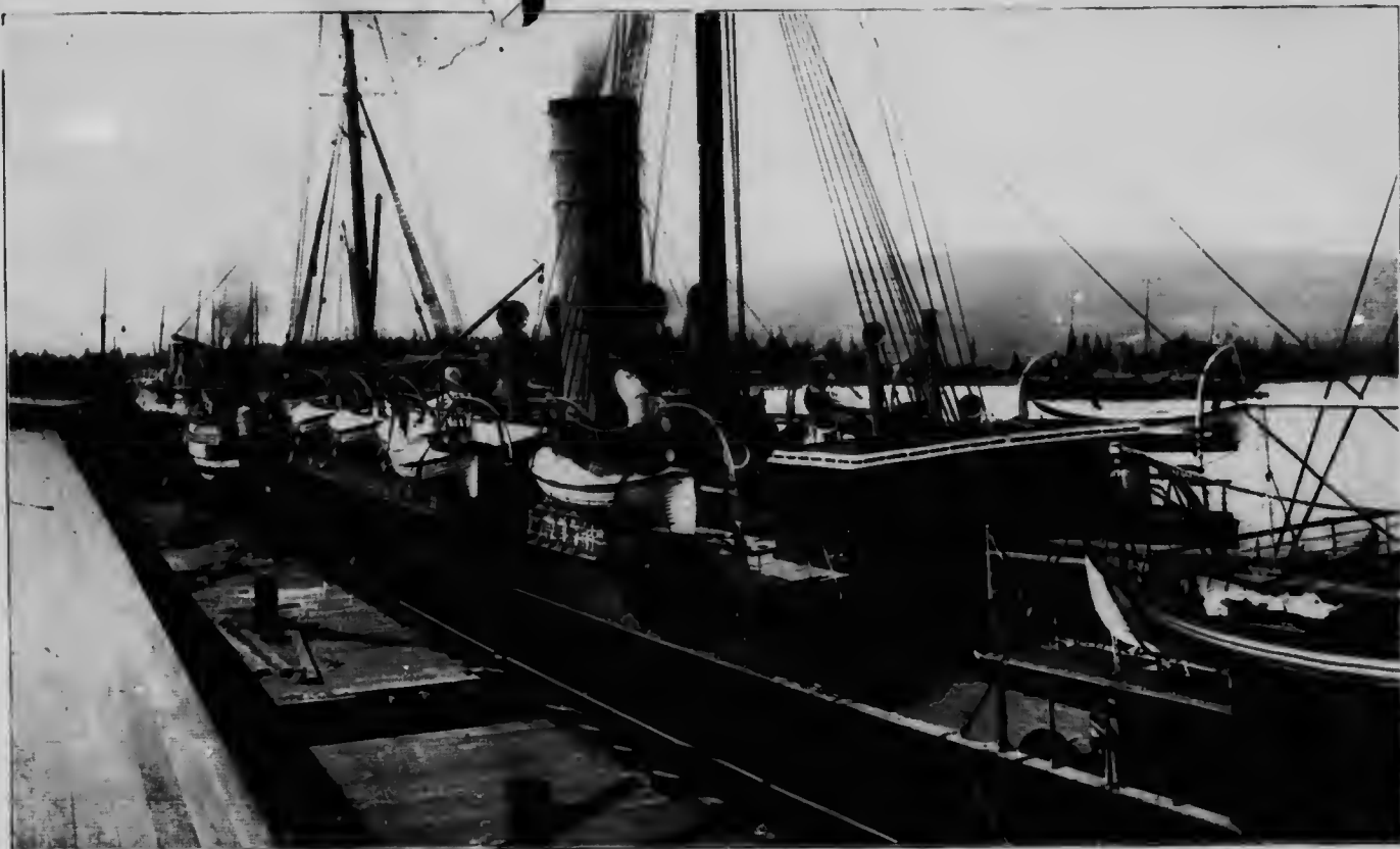
PORTION OF TRANSPACIFIC DOCK, VANCOUVER, B. C.
