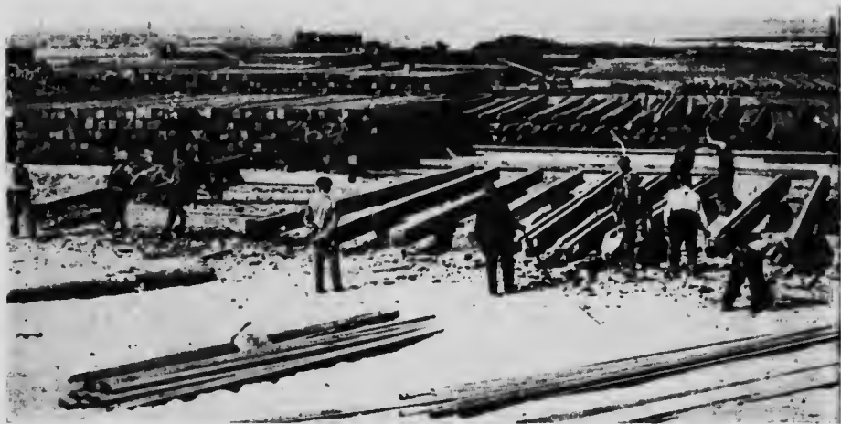
Douglas fir timbers for use in Toronto harbour construction. Nineteen million feet, board measure, of Douglas fir are being used in this work.
