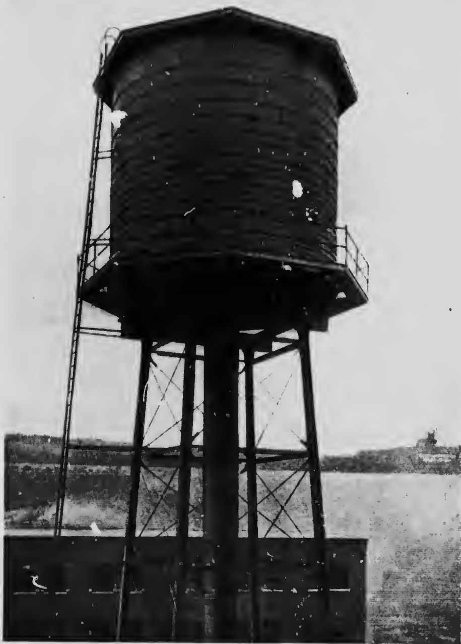
A fifty thousand gallon water tank built of red pine, Montreal. Red pine is the best Eastern Canadian wood for this purpose.
