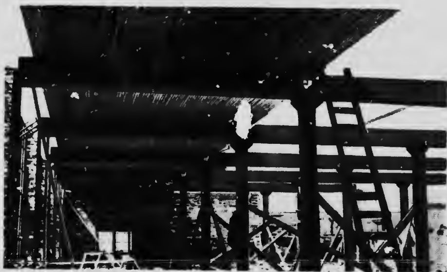
Mill construction, showing timbers and laminated flooring, two very important uses for Douglas fir.
