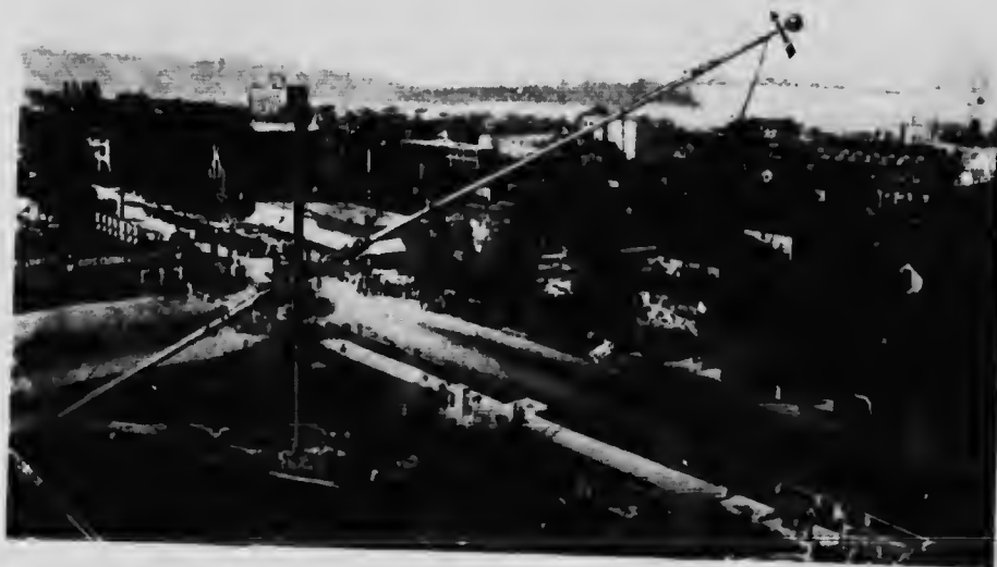
Flagpole being erected in front of Court House, Vancouver, B.C. This is a single stick of Douglas fir 210 feet long.
