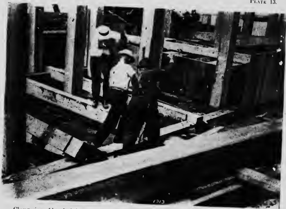
Closer view of hemlock in Toronto harbour construction. Seven million feet, board measure, of this wood are being used in this work.
