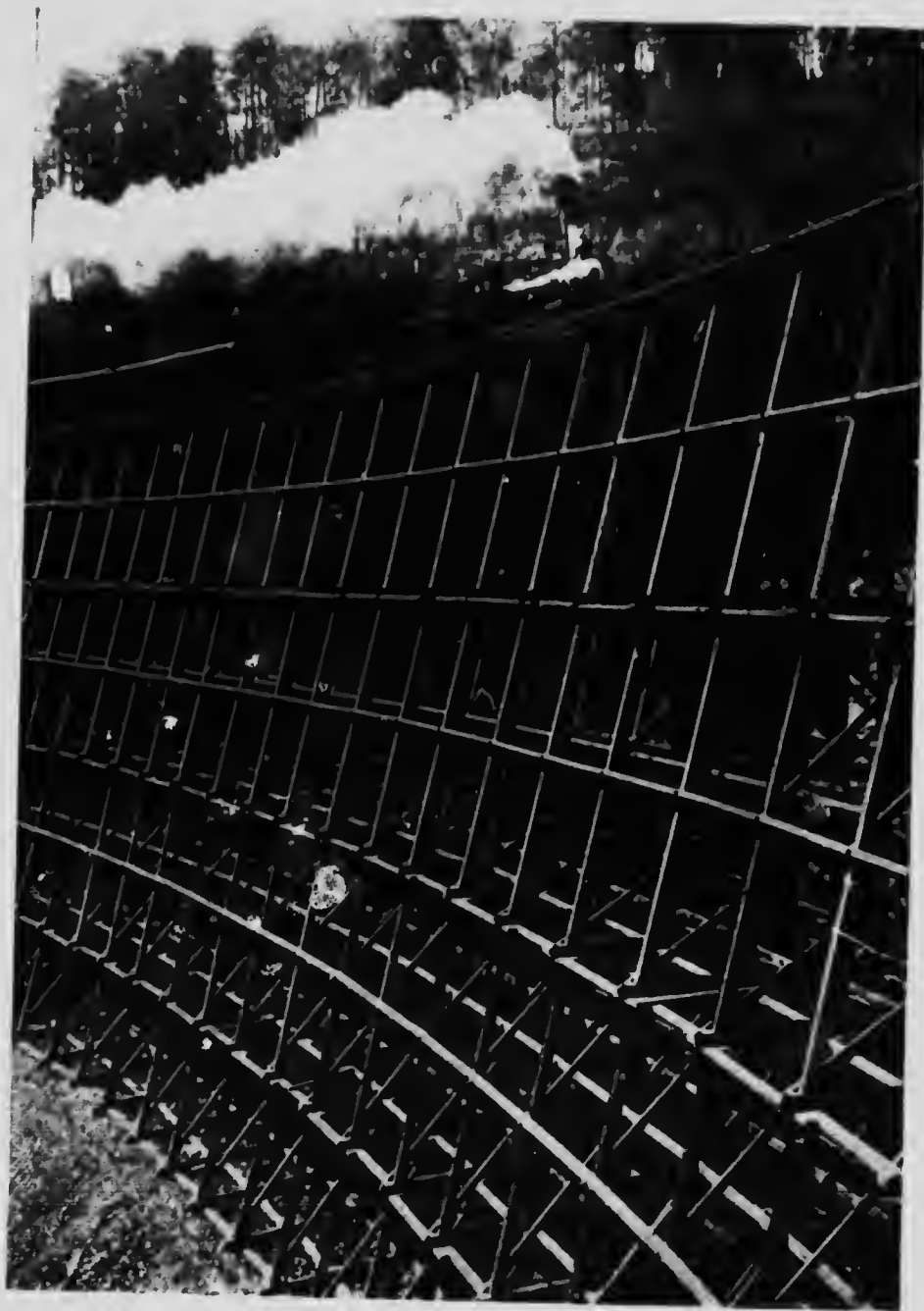
Bridge trestle on the Canadian Pacific Railway, built of Douglas fir in 1896. 10882—31
