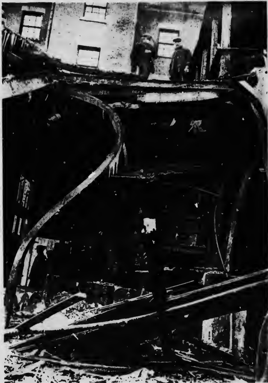
View after a fire in a factory in Montreal. Note steel work twisted and useless while timber is still in place and supporting a load.
