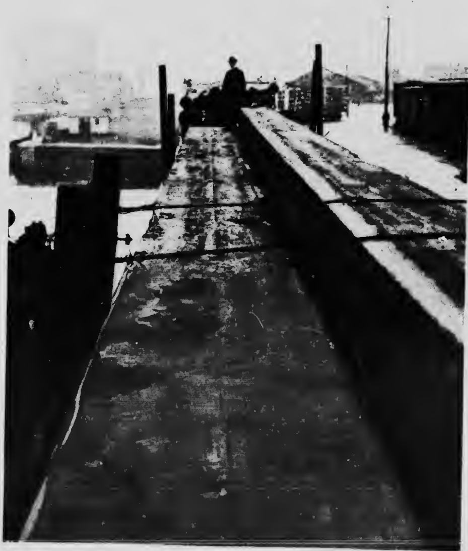
Another view of the big Douglas fir timber 46 by 46 inches by 70 feet, for use in Montreal harbour work.
