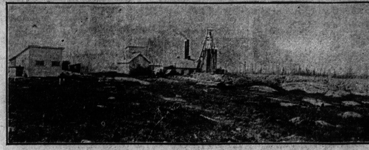
Showing headframe and plant of West Dome Consolidated Mine.
