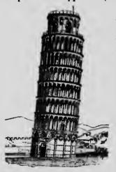
Fig. 53.—The Leaning Tower of Pisa. It overhangs its base more than 13 feet, but it is stable. (Drawn from a photograph.)
