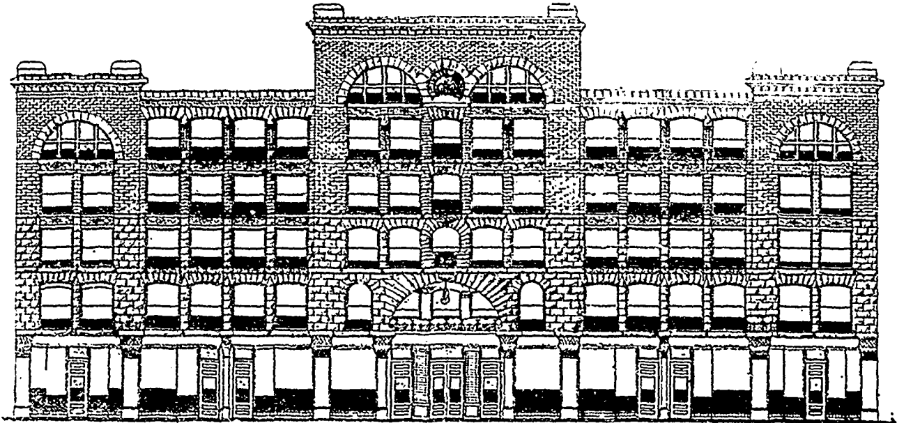
Handsome New McIntyre Block Building, Main Street, Winnipeg, now Nearing Completion.
