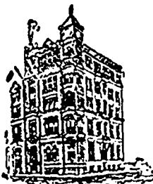
HEAD OFFICE BUILDING, MONTREAL.
