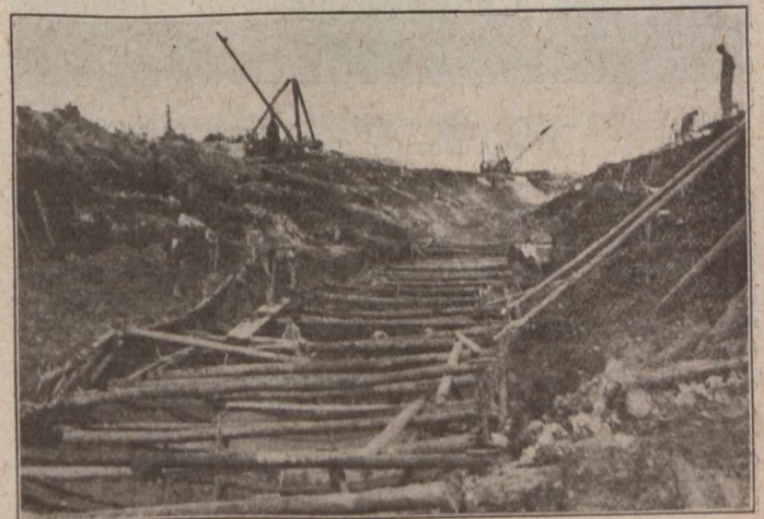
FIG. 6—SHEETING THROUGH SLIDE
