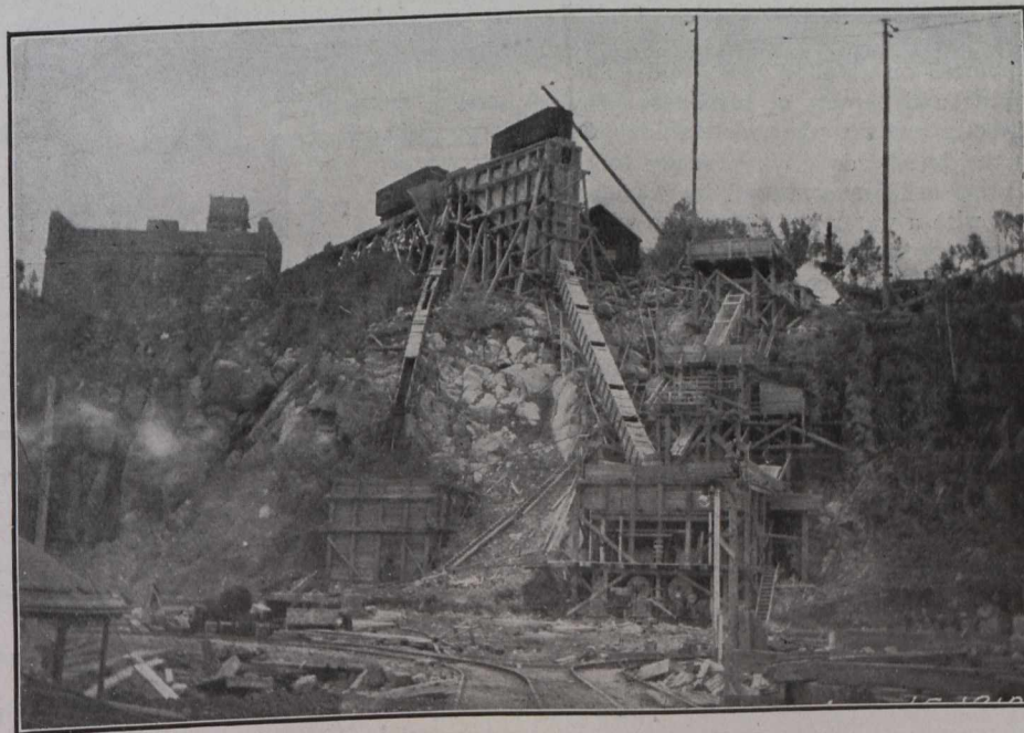
The Plant on the Side of the South Cliff.
