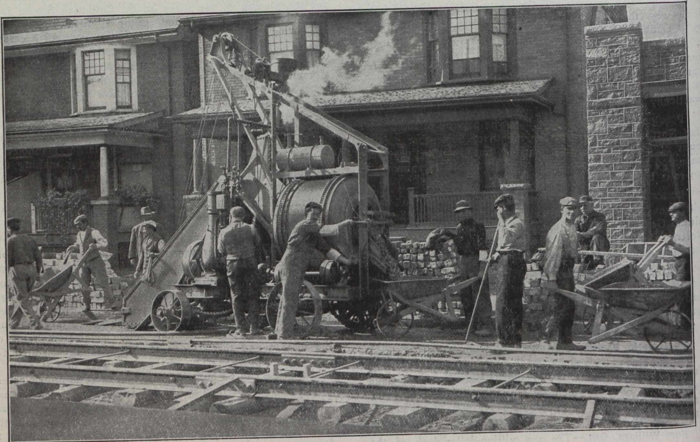
Placing Concrete on Foundation for Civic Car Lines, Toronto.
