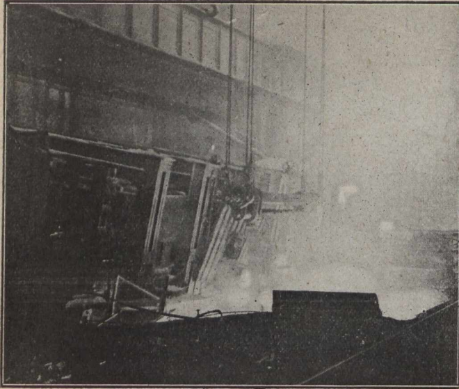
Tapping a 50-Ton Furnace.
