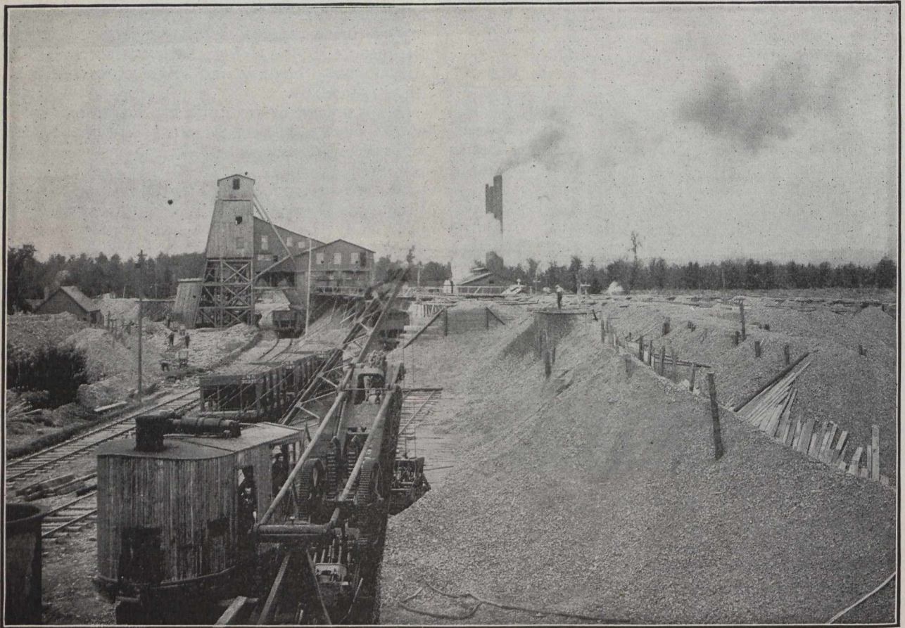
Torbrook Surface Plant
