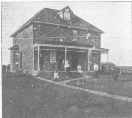
View of residence of A. B. Potter, Montgomery, Sask.
