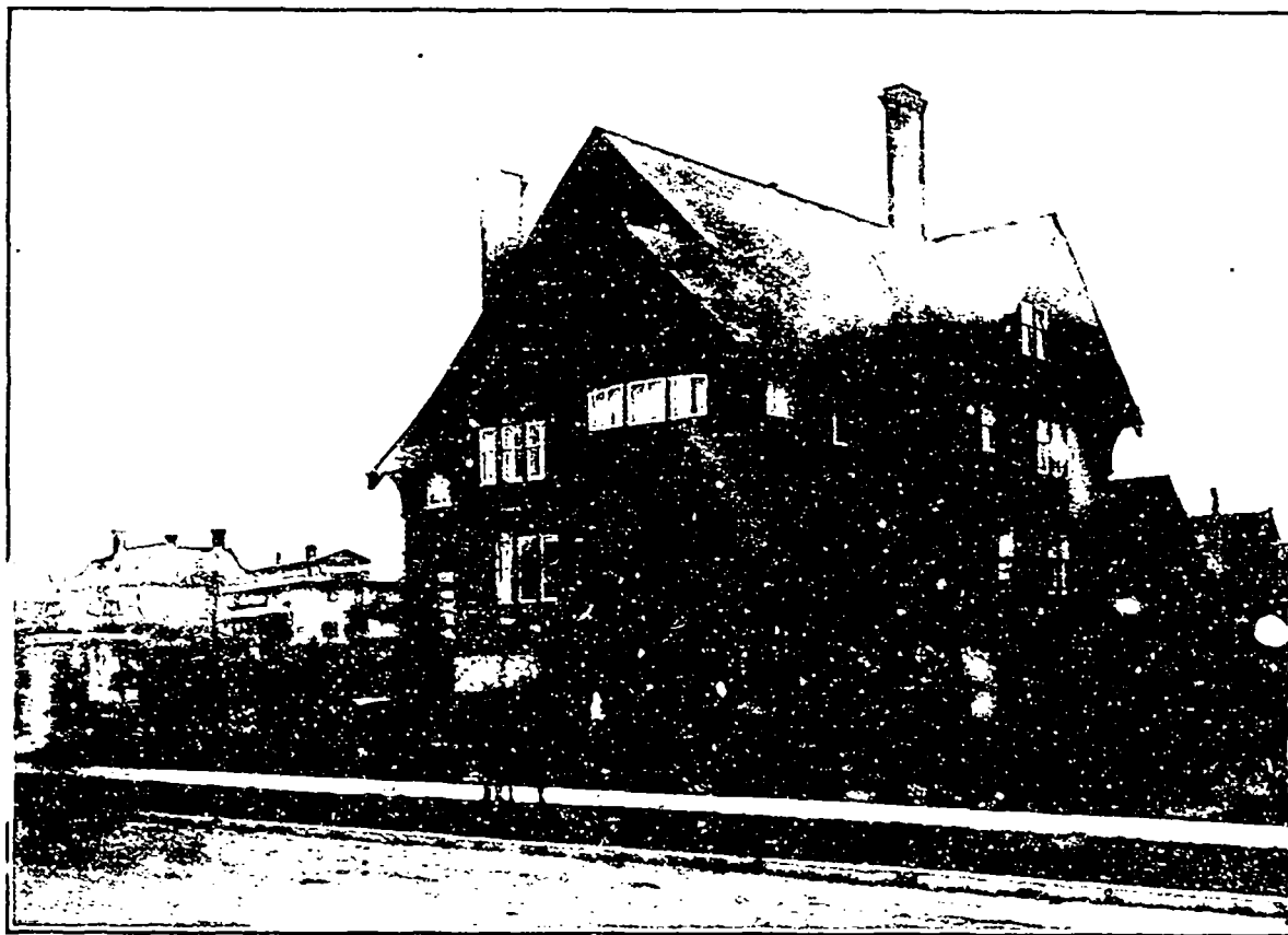
RESIDENCE OF MRS. L. I. DISSETTE SHAUGHNESSY HEIGHTS VANCOUVER, B. C.
