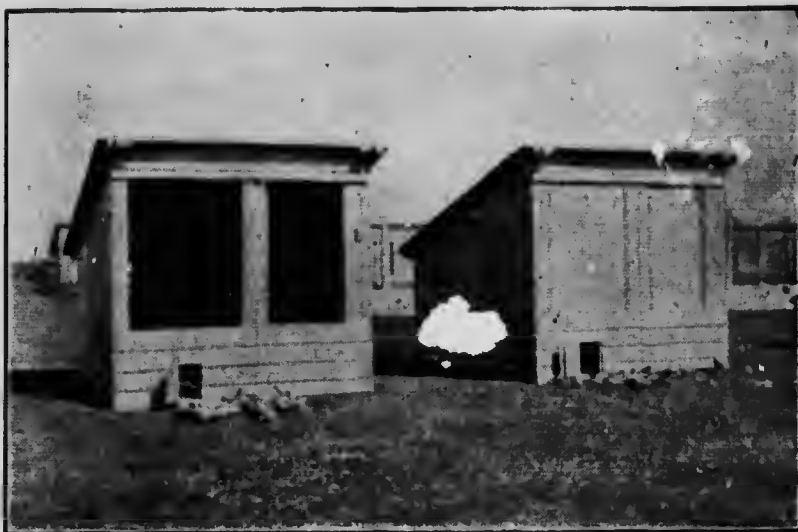
FIG. 31.—A STYLE OF BROODER HOUSE EXTENSIVELY USED AT THE PROVINCIAL STATION.
