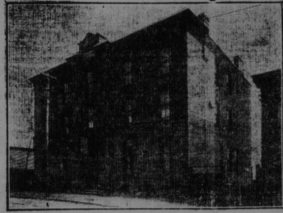
People's Palace, St. James Street. Renovated at a cost of $5,512.07, and being re-equipped for better service.
