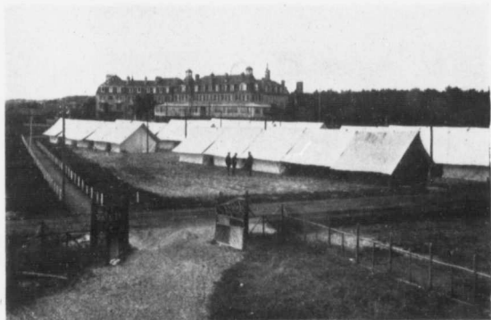
VIEW OF NO. 2 STATIONARY HOSPITAL —SOMEWHERE IN FRANCE.
