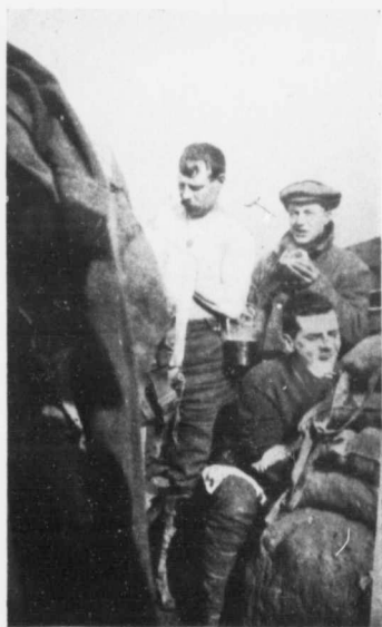
A TRENCH TOILET—AT THE FRONT.
