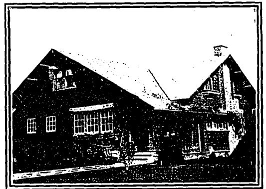
DESIGN NO. 10.—A CLAPBOARDED ONE STOREY AND A HALF BUNGALOW WITH SMALL CORNER PORCH. THE DESIRED EFFECT IS PRODUCED IN THIS DESIGN THROUGH THE BROAD OVERHANGING ROOF, THE OUTSIDE CHIMNEY, THE WINDOWS AND THE COLOR SCHEME.—F. G. BROWN, ARCHITECT.
