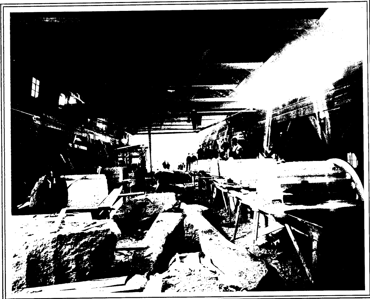
MAIN WORK SHOP AT QUARRIES AT STANSTEAD, P.Q., SHOWING CUTTERS WORKING ON THE 13-TON DRUMS FOR THE COLUMNS OF THE BANK OF COMMERCE, MONTREAL.
