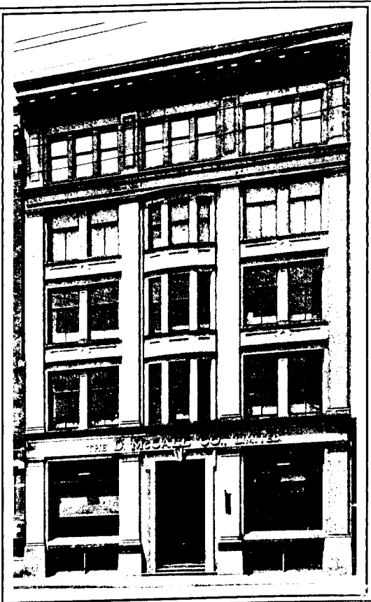
THE McCALL WAREHOUSE WELLINGTON ST. WEST, TORONTO GEO. W. GOUNLOCK, ARCHITECT
