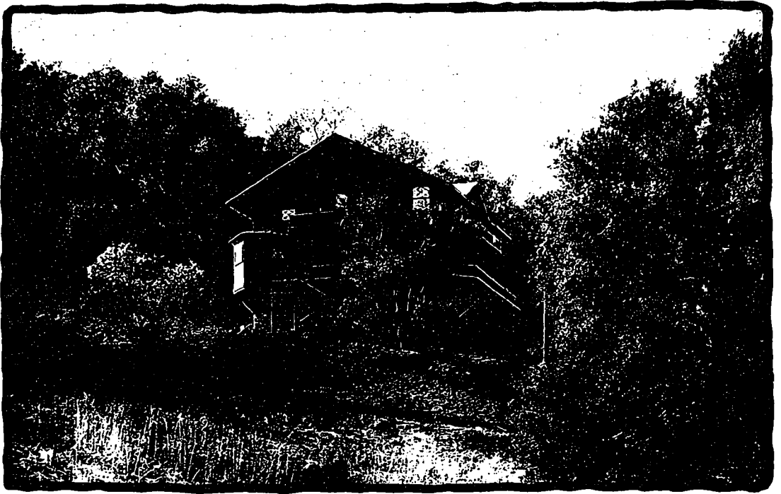
DESIGN NO. 1.—SWISS CHALET OF MRS. WILLIAM MARVIN OF SOUTH PASADINA, CALIFORNIA. F. G. BROWN, ARCHITECT. IN DESIGN, PLAN AND SETTING THIS IS AN IDEAL OF THIS POPULAR MODIFICATION OF THE PRIMARY BUNGALOW THAT HAS GAINED GREAT FAVOR IN BRITISH COLUMBIA, AND IN THE SUMMER RESORTS OF EASTERN CANADA. ITS BROAD OVERHANGING ROOF, CRUDE PORCHES AND RUSTIC HUE TEND TO MAKE THE BUILDING A VERY PART OF ITS PICTURESQUE SURROUNDINGS. THIS STYLE OF BUILDING IS BEST SUITED TO A SITE ON THE SIDE OF A HILL WHERE IT CAN BE MADE TO HARMONIZE MORE EFFECTIVELY WITH ITS SURROUNDINGS THAN ALMOST ANY OTHER FORM OF BUILDING.
