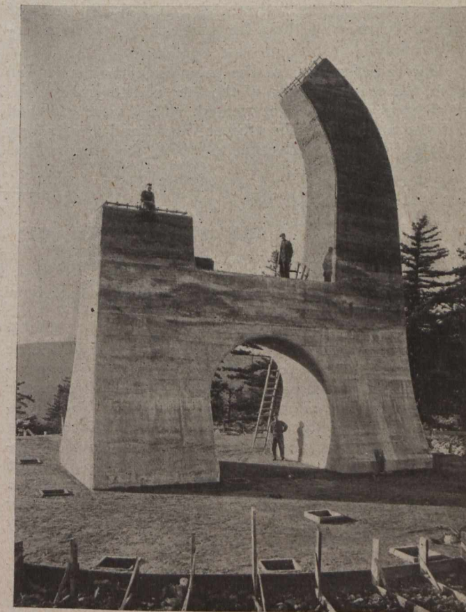
Telescope Pier and Telescope Building Foundation.
