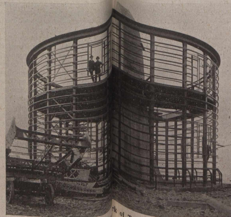
Structural Steel Framework of Telescope Building.
