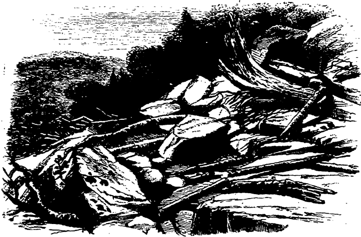
LAND-SLIDE ON COLD-WATER RIVER PORTAGE.
