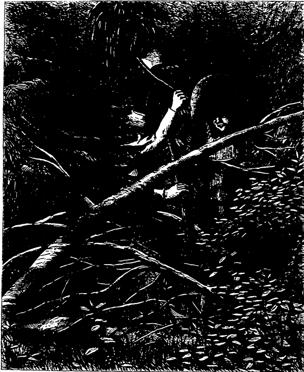
CUTTING OUT A ROAD.
