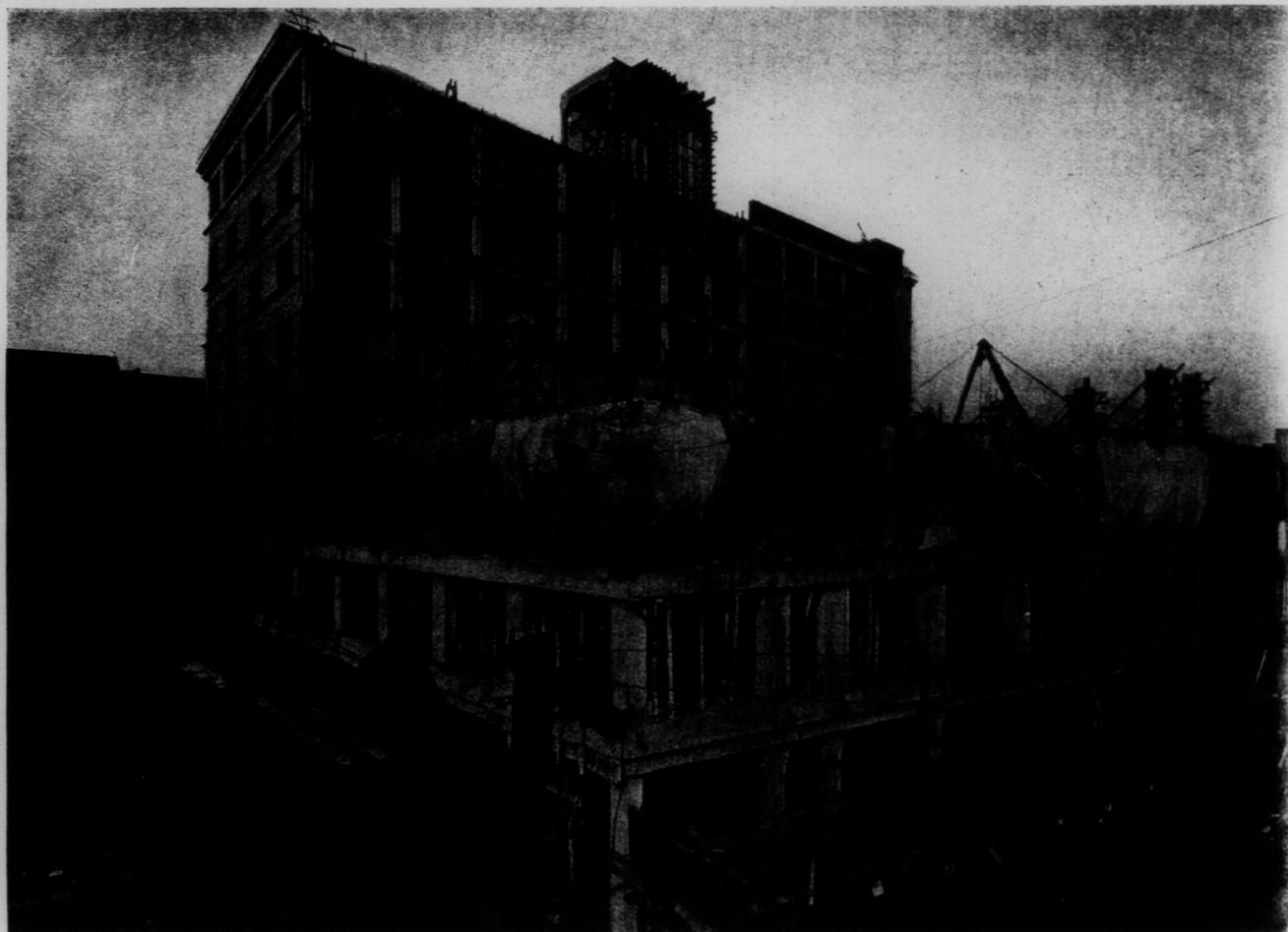
ACME TEA CO.'S WAREHOUSE—SHOWING STEEL AND CONCRETE CONSTRUCTION.
