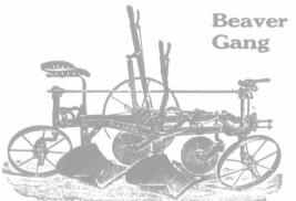
Furrow and rear wheels are connected and controlled from the pole. By this arrangement the plow is easily guided when working or turning at the ends.
