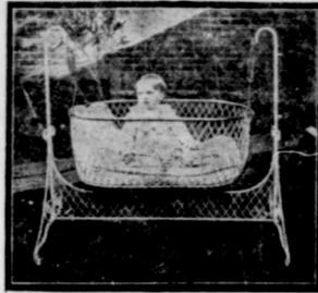
NOTE Double springs attached to the bassinette hang from the standards and respond to the slightest movement of the child.
