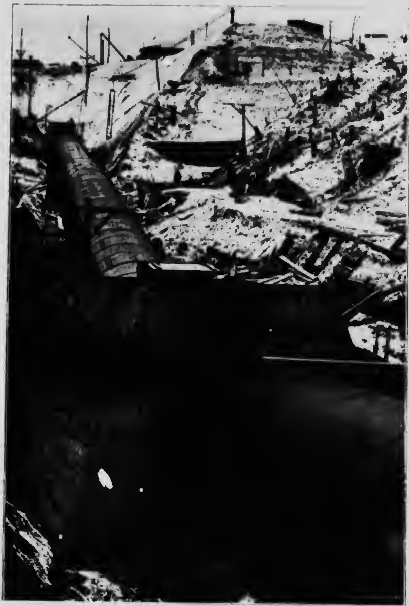
One of the Pen-stocks that feed the Pulp Mill during construction
