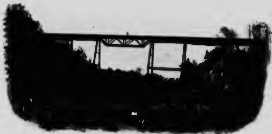
St. Clair Bridge
