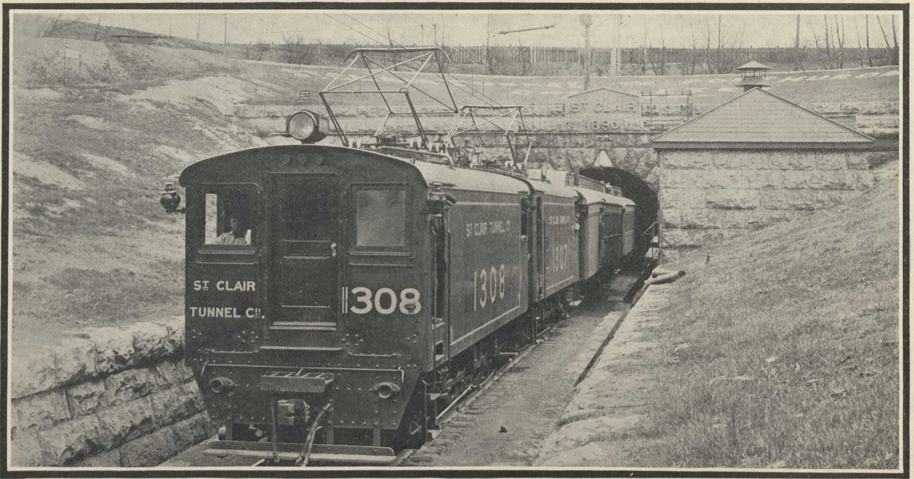
A Double Electrical Locomotive drawing a train out of the St. Clair Tunnel. This double engine will draw a train of 1,000 tons up a two per cent. grade at a rate of more than 10 miles an hour. The use of electricity has quadrupled the capacity of the Tunnel.
